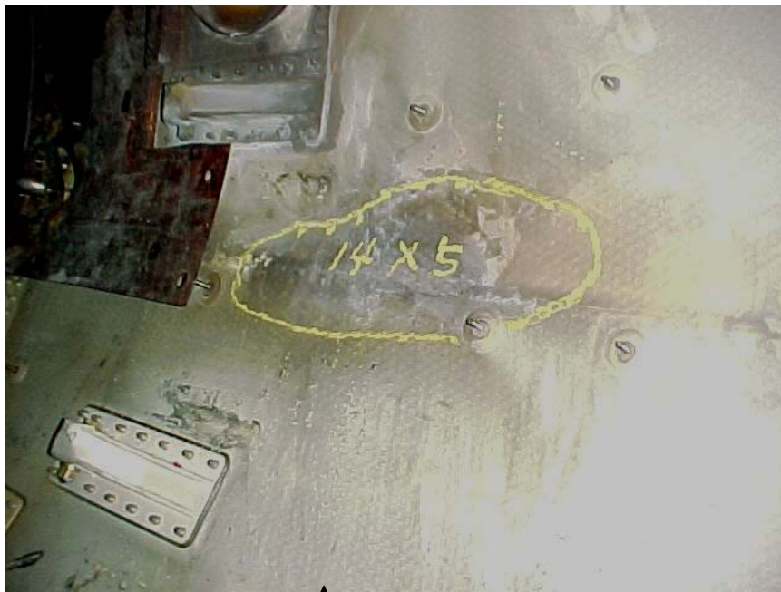
Overheat Damage at Blanket Seam
